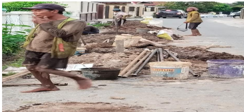
Figure 1. Excavation work on Jl. Arjuna, RW 08 and 09, East Labuh Baru, Pekanbaru
